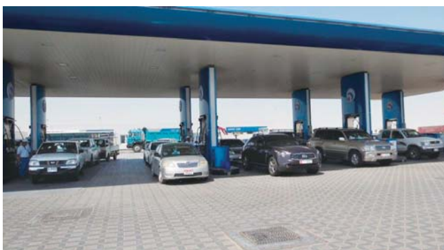
Fueling island at SS949 (photo provided by JX Nippon Oil & Energy Corporation)
