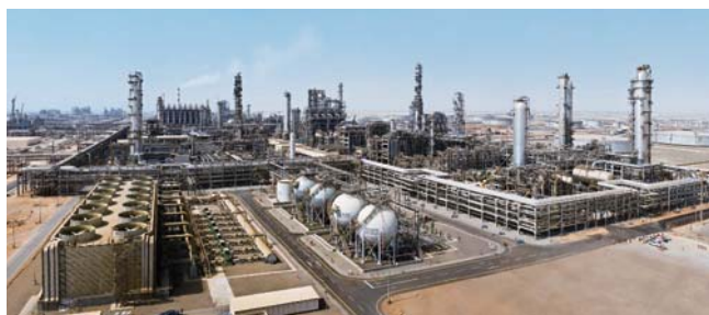
PetroRabigh Petroleum Refining and Petrochemical Complex (photo supplied by Saudi Aramco)
