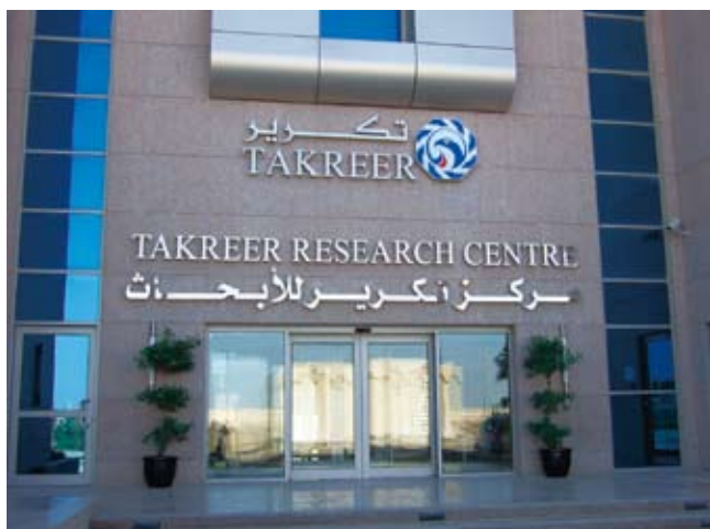
The completed TAKREER Research Centre
