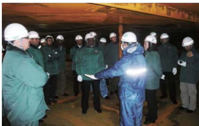
Inside a crude oil tank open for inspection
