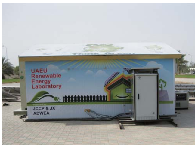
Fuel cell housing structure
