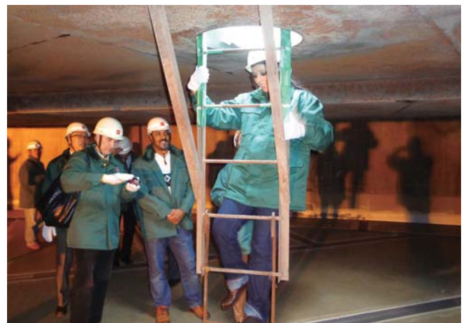
Inspection of a 100,000kL crude oil tank that is open for overhaul
