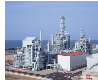
500BPSD GTL Demonstration Plant Chiyoda's CO 2 Reforming Process is used for synthesis gas production in National GTL project by JOGMEC and Nippon GTL Technology Research Association.
