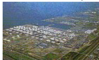
Chiba refinery and petrochemical plant
