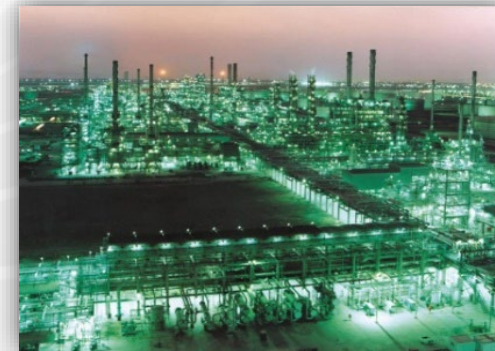
MINA ABDULLAH REFINERY 454 KBPD
