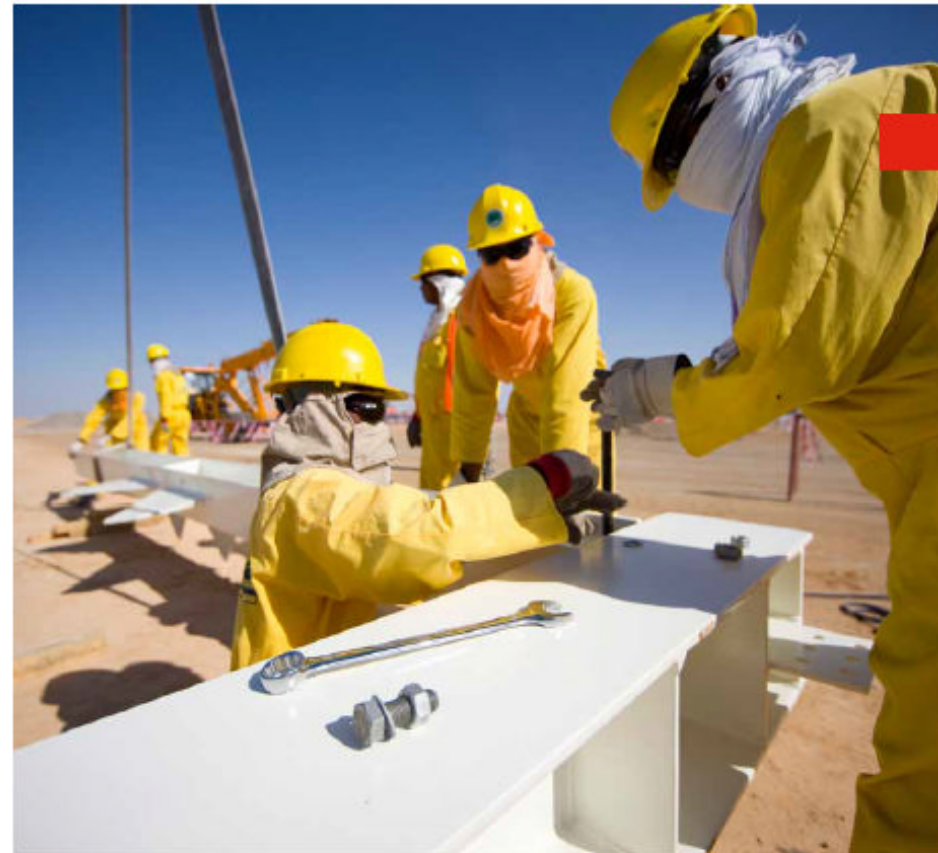
Construction at the Qarn Alam EOR project, Oman
